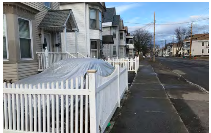
Cars are frequently parked in front yard areas between Brandywine Avenue and Steuben Street.
