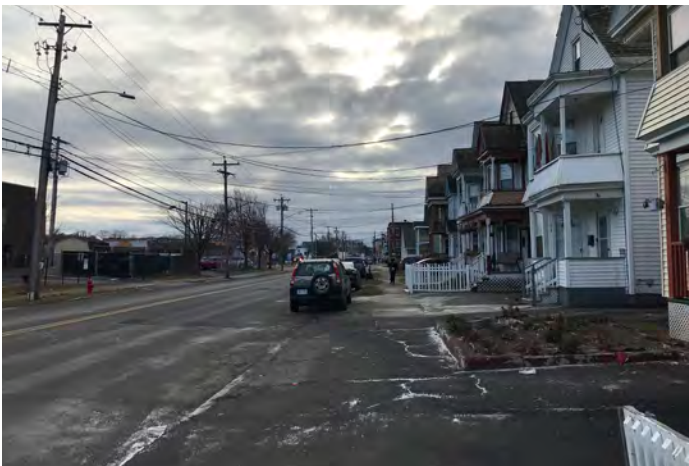
There are many areas along the Albany Street corridor where the curb is barely evident and the sidewalks have been paved over with asphalt. Tree lawns have also been paved over and this, in combination with the absence of street trees, has led to cars regularly parking in the tree lawn and on the sidewalk. This photo was taken on Albany Street between Brandywine Avenue and Steuben Street.
