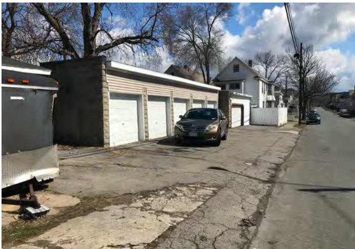
Portions of the sidewalk have been paved over with asphalt. In the instance above, this long garage prohibits on-street parking and preferences vehicular use over pedestrian travel.
