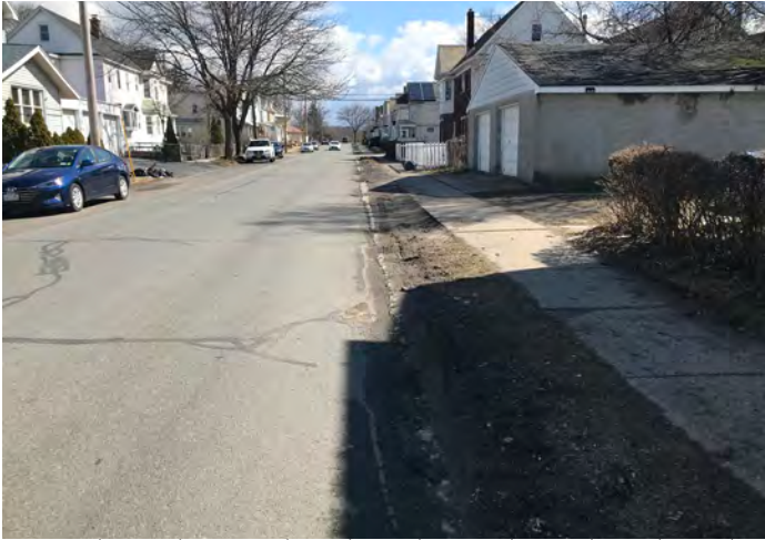
Tire tracks can be seen throughout the tree lawn where the curb is almost gone and cars routinely drive and park.
