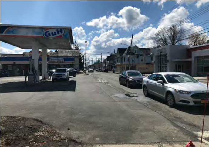
The absence of a curb and sidewalk on the Crane Street side of the Crane / Main / Chrysler intersection gas station equates to a 130 foot curb cut, allowing cars to enter and exit the site anywhere along that stretch, including very close to the intersection. This also makes it much more challenging for pedestrians.
