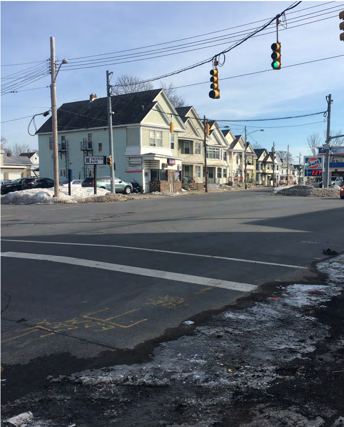
The Crane / Main / Chrysler intersection has a high concentration of accidents involving bicycle users and pedestrians. As seen here, there are few pedestrian accommodations and most of the crosswalk striping is either worn away or missing.
