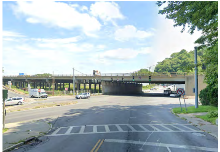
Pedestrian and bicycle options for navigating the Crane and Broadway intersection are extremely limited and require first going in the opposite direction that is desired.
