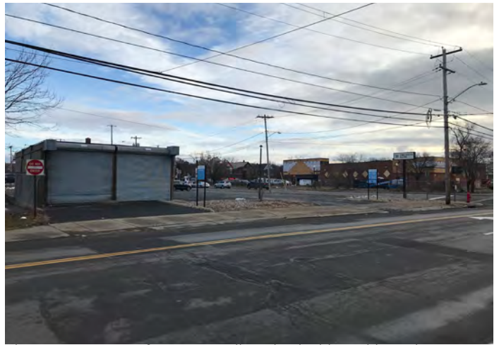
There is no sense of a street wall at this highly visible and important northern corner of Albany Street and Brandywine Avenue where the lot is occupied by parking and contains no street trees. This situation likely contributes to higher speeds on Albany Street. The absence of trees also calls greater attention to the unsightly overhead utility lines,
