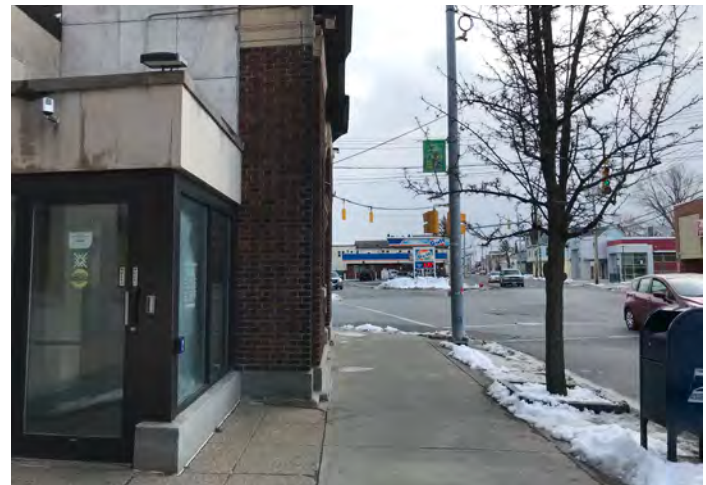
Some portions of the sidewalk have pavement that is in relatively good condition and there are a few street trees along the corridor to the north of Main Avenue.
