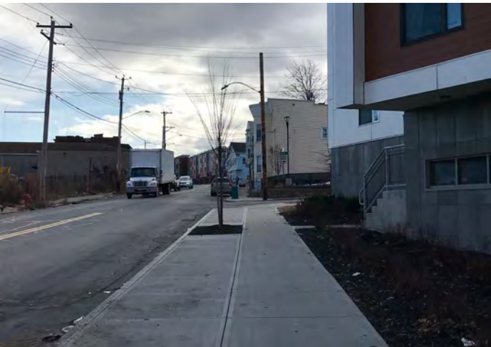
The three mixed-use affordable housing developments between Craig Street and Veeder Avenue each include new sidewalks, full size curb reveals, and street trees.
