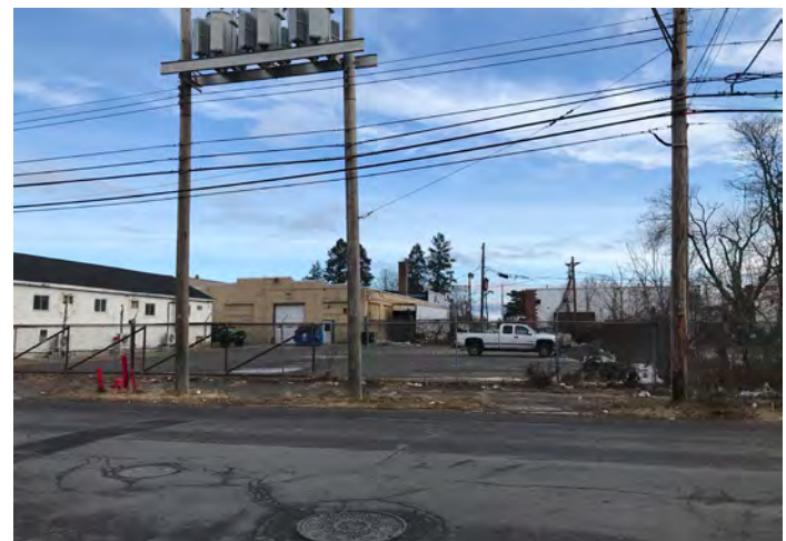
The abundance of large parking areas with no tree cover greatly adds to the urban heat island effect, limiting the ability of the area to cool at night and making it much hotter during the day. This situation is an example of the disadvantages faced by environmental justice communities.
