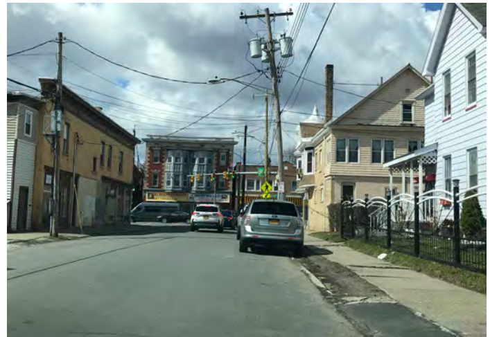
Cars frequently straddle the curb on Francis Avenue. In many locations, the road is higher than the curb and the tree lawn fills with ponding during storm events.
