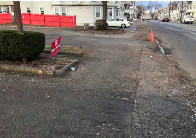
Non-existent curbs and uninterrupted asphalt detracts from the walkability of the street and encourages detrimental parking habits. This photo was taken on Albany Street between Brandywine Avenue and Steuben Street.
