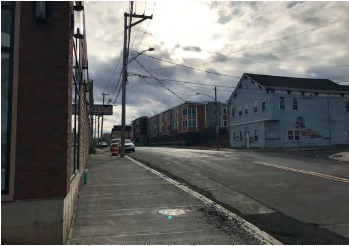
In some areas, the curb and sidewalk have been replaced, but the sidewalk remains narrow and there are no street trees or vertical barriers to increase pedestrian safety and calm traffic. This photo was taken between Craig Street and Veeder Avenue.
