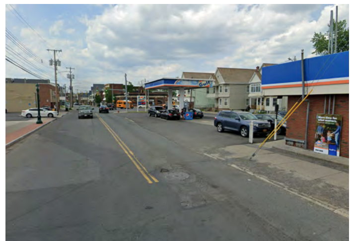
The sidewalk on the east side of Crane is missing in the south area closest to the Main / Crane / Chrysler intersection, which makes walking more challenging, encourages higher speeds, and adds to the general confusion in the area of the intersection..
