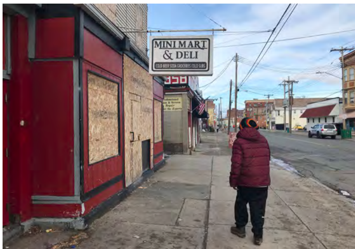
Many of the curbs are at or below street level as seen in this photo taken between Steuben Street and Craig Street.
