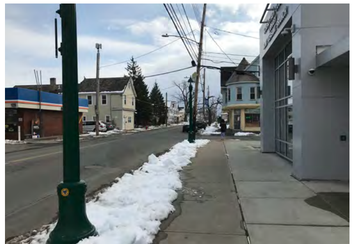
The new Mont Pleasant Library branch includes new sidewalks and higher curb reveals, but unfortunately no street tree and few vertical barriers between the roadway and the sidewalk.
