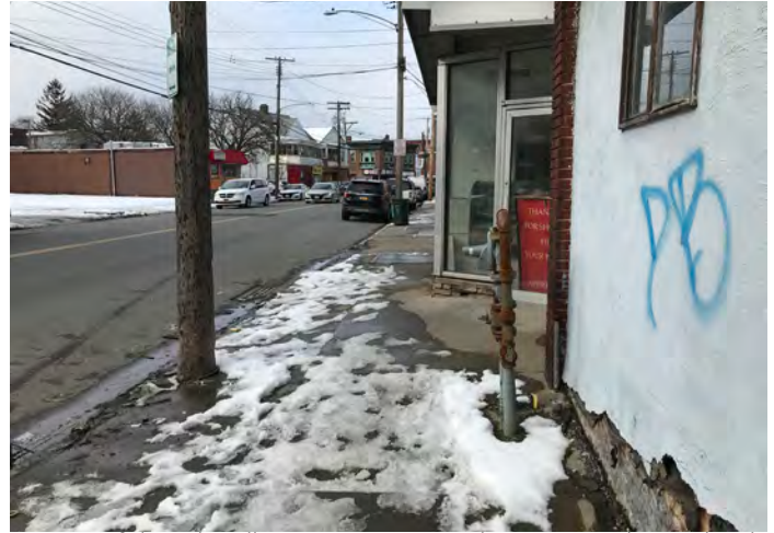
Portions of the sidewalk are very narrow and sometimes cluttered with utilities. This photo was taken between Main Avenue and Francis Avenue.
