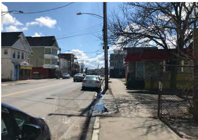
In some places, the road is higher than the absent curb reveal, leading to ponding along the sidewalk. This photo was taken between Main Avenue and Francis Avenue.
