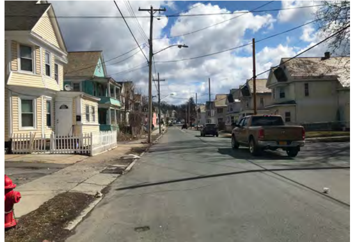
Much of the curb reveal on Forest Road and Francis Avenue is missing. There are also very few street trees. Sidewalks tend to be in better condition than surrounding streets, but several show signs of spalling, heaving and breaking, particularly at driveway locations.
