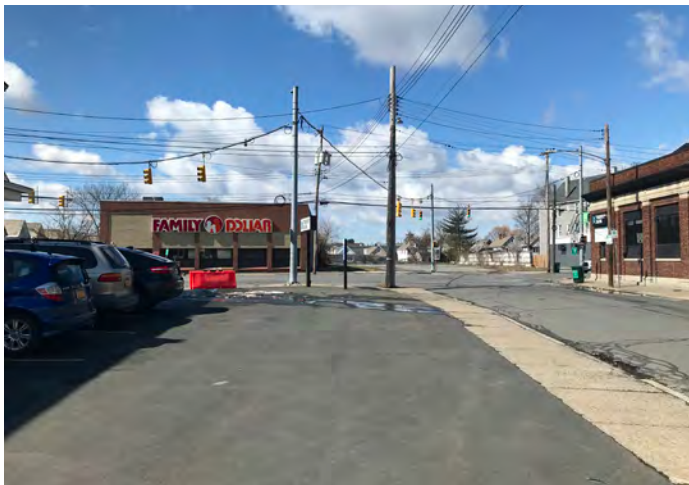
The parking lot at the Crane / Main / Chrysler intersection has a low to zero curb reveal, which functions as a 170' curb cut and encourages cars to back into the road at points very close to the intersection. It is also lacking in any vertical elements that could help with traffic calming and enhancing the pedestrian experience.
