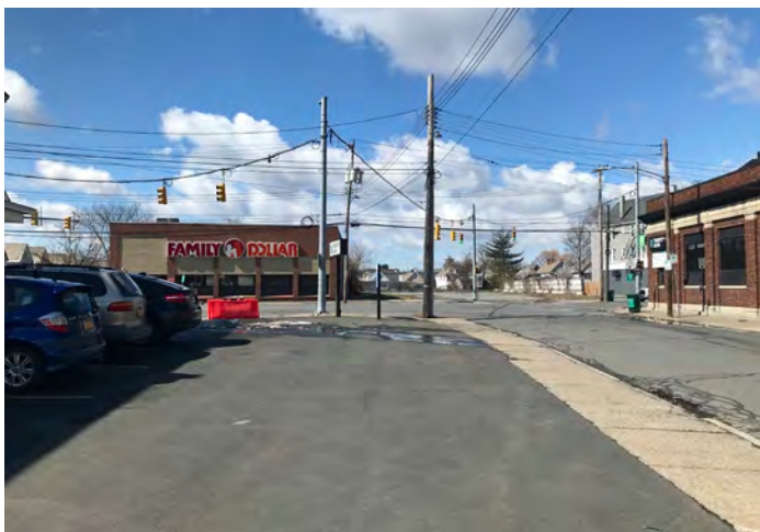
The sidewalk closest to the Crane / Main / Chrysler intersection doubles as a vehicular use area where there is no curb reveal and cars back over it to enter and exit the parking area.
